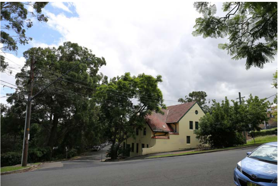
Existing view from Beaconsfield Parade
